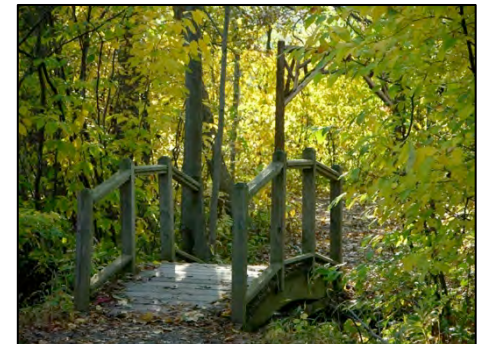
Above (top to bottom): View of Esopus Creek from the Saugerties Light House; view looking across Esopus Creek looking west toward Catskills; and view of walking trail pedestrian bridge (photos courtesy Joy Moore). The Town/Village of Saugerties natural resources help to define the community and enhance the quality of life.
