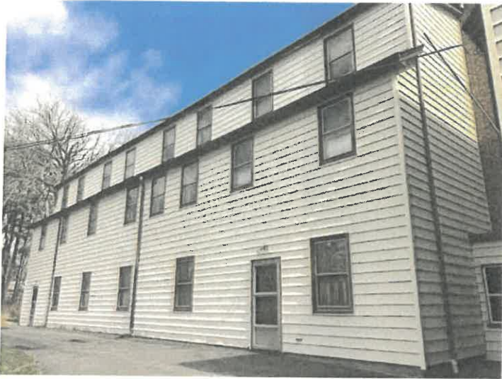
Photo 5. The northern portion of the west elevation of Villa St. Joseph.
