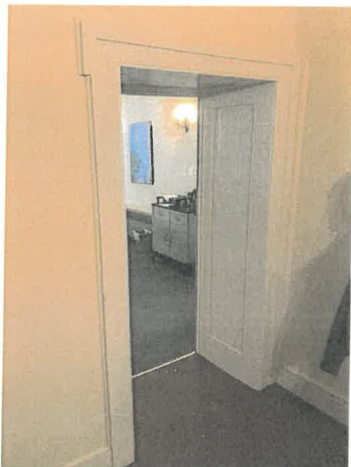
Photo 17. From within Section B, looking east to the dining room in Section A. The doorways of Section B have shouldered surrounds. The wall between Section A and Section B is thick, suggesting the stone construction of Section A.
