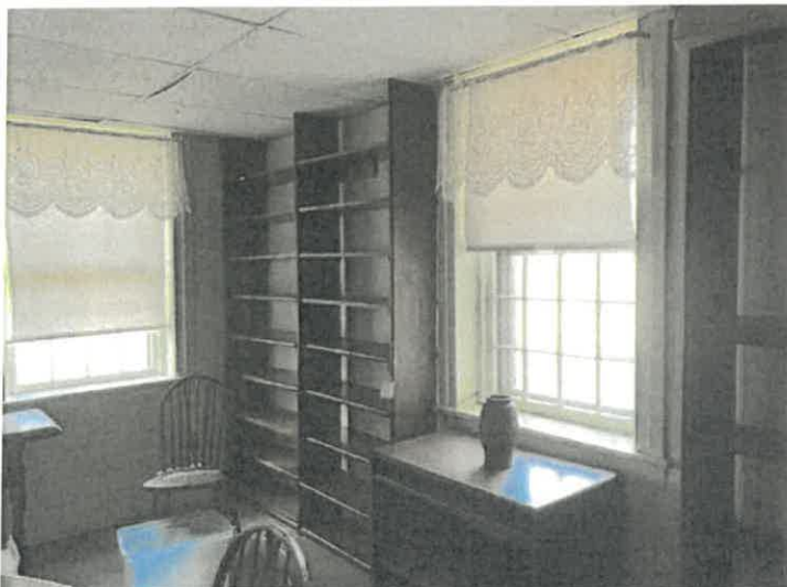
Photo 20. One of the rooms on the first story of Section B. While largely remodeled, the room retains windows with twelve-over-twelve-light wood sash.
