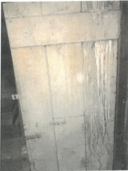
Photo 28. A batten door in the basement of Section A.
