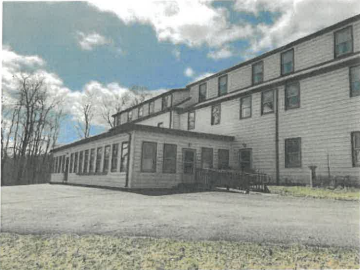
Photo 3. Another view of the east facade of Villa St. Joseph.
