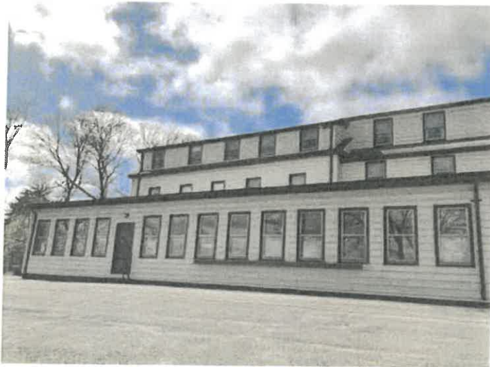
Photo 2. The east facade of Villa St. Joseph.
