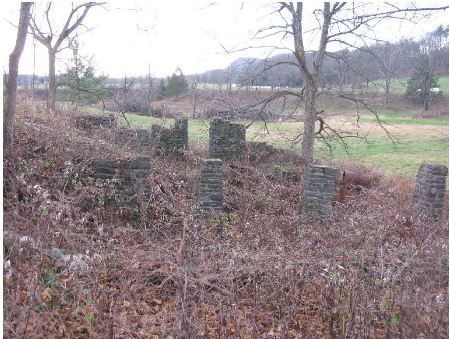
Photograph 9. Barn foundation with central pillar supports (#3). View southwest.
