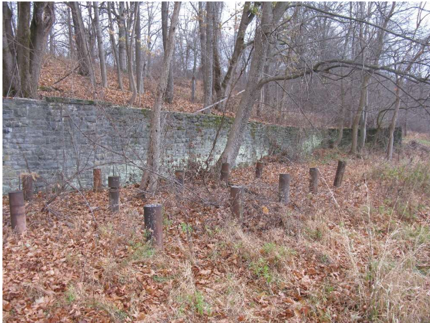
Photograph 10. Undetermined structure with iron pier supports and long bluestone retaining wall (#4). View northwest.
