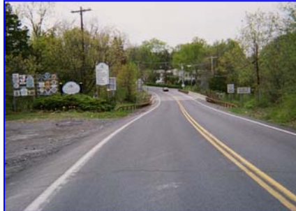
Existing view of bridge near Seamon Park
