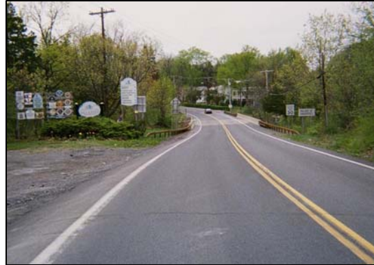
Existing view of Route 9W at the Sawyer Kill bridge.
