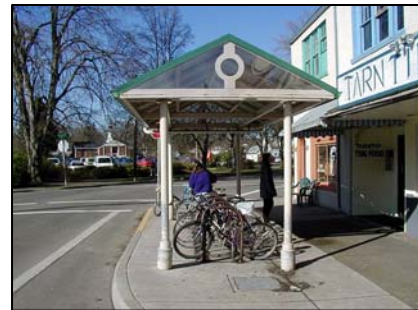
Example of covered bike rack.
