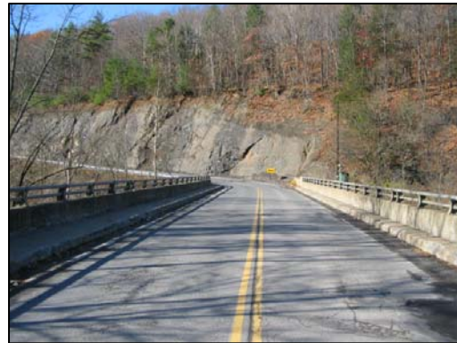
Bridge over Esopus Creek (B.I.N. 3346850) and rock face on far side.
