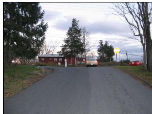
View of Krout Road upgrade
